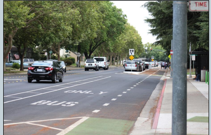
Roadway with Bus lane, Bus Stop and Class I Bike lane in Modesto
