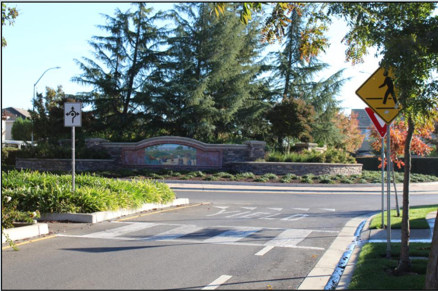
Traffic Circle/Roundabout and Pedestrian Crossings
